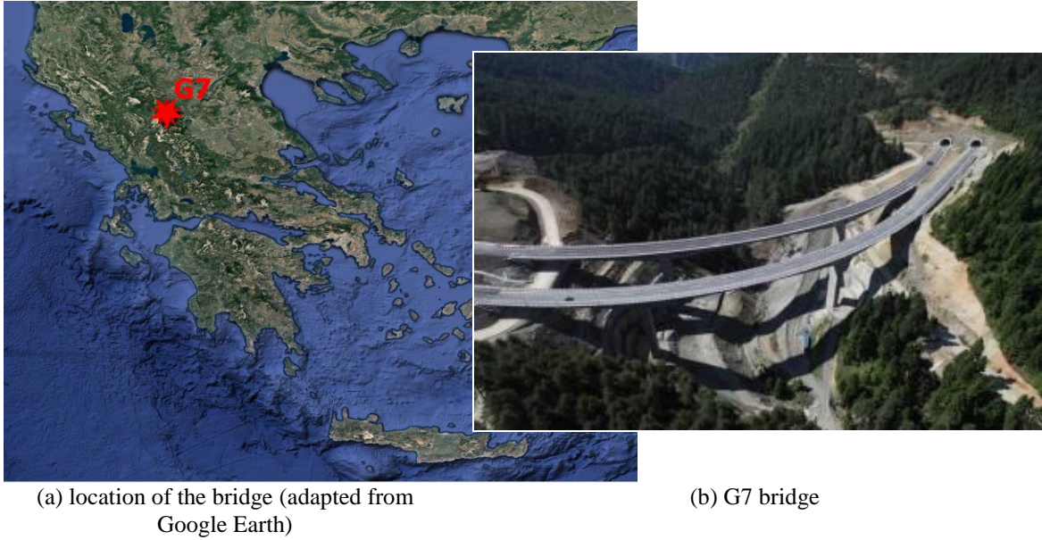
Fig. 2 – G7 bridge of the Egnatia Odos highway in Greece.
